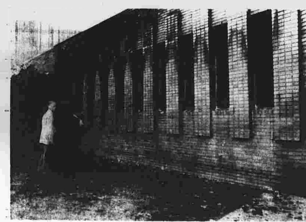
West Hartford authorities check the scene of Monday's arson fire which damaged the Emanuel Synagogue, the second West Hartford synagogue damaged by fire in a week. Police believe the same person is responsible for both fires.
